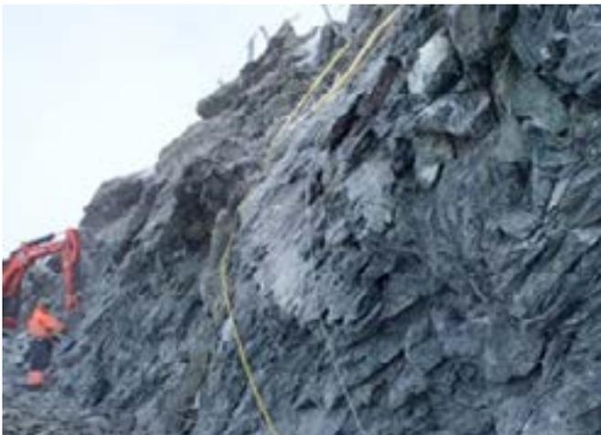
Strongly foliated serpentinite at the excavation front. (b) Typical superficial undulated rock flakes
